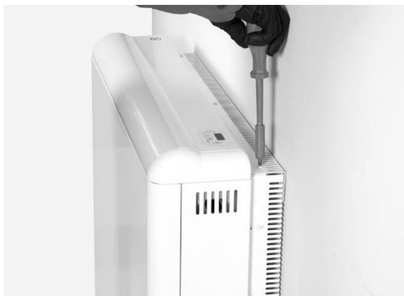
**ECOHR MUST NOT BE HUNG ON THE SCREWS;** these are used only to prevent the device from overturning and not to support it. If there is any doubt concerning the wall strength, consult the corresponding construction specialist. The appliances are heavy; it is the installer responsibility the correct installation and wall support of these devices to prevent them from overturning.
