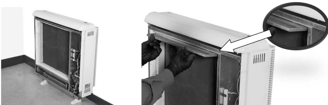
10. - Place the second row of storage bricks with the flat side facing out.
