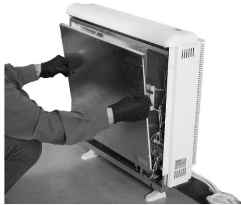
8. - Do not disconnect the electrical heating elements. Remove the packing cardboard and the metallic part. Lift and tilt the elements outwards being careful not to damage the insulation on the bottom of the heater and place carefully the storage bricks. Arrange two levels of bricks with the flat side facing the back of the heater.
